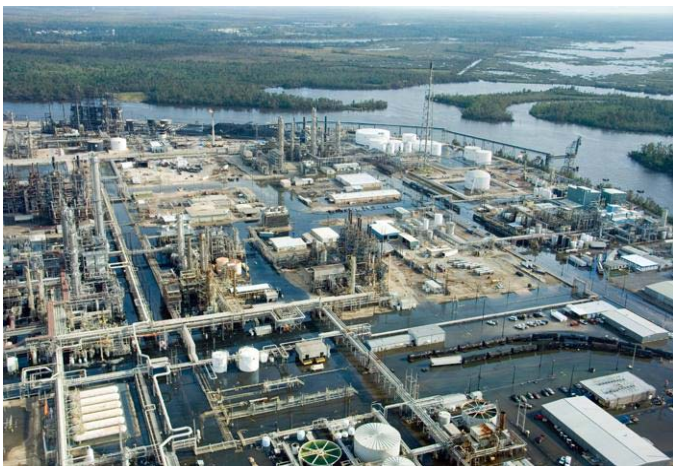
Figure 19. Flooded refinery near Beaumont, Texas, in the aftermath of Hurricane Ike
