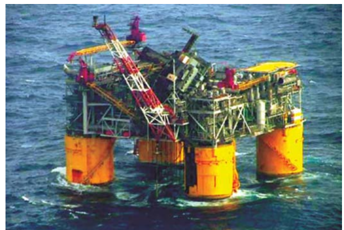
Figure 20. Damaged offshore platform after Hurricane Katrina
